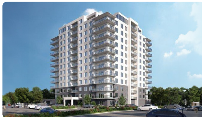
Realstar building on Brookline Drive in Bedford, NS
